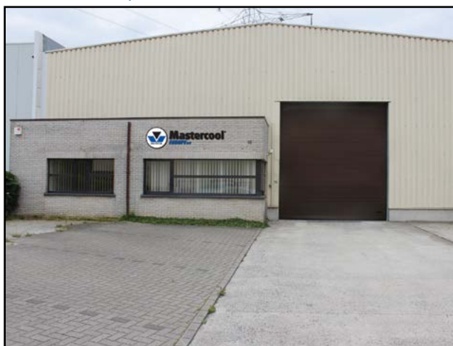
European Sales Office and Warehouse
